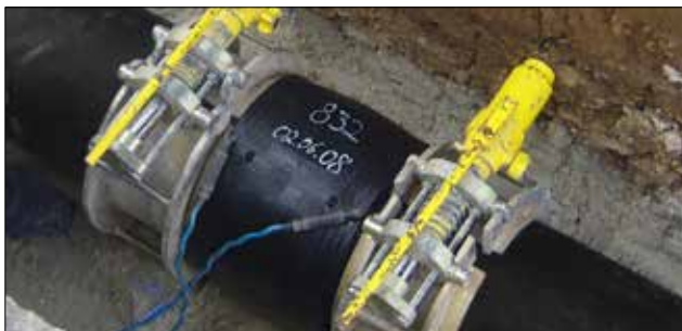
8.49 Re-rounding clamps for EF joints (source: +GF+)
