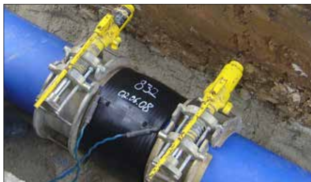
6.81 Re-rounding clamps for EF joints (source: +GF+)
