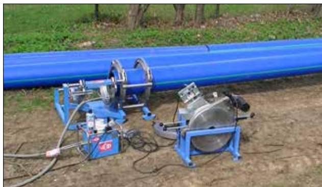
6.26 Gerodur service: provision of project-specific clamps for butt fusion (Widos) – delivery in robust heavy-duty box
