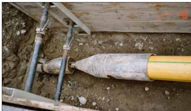
6.25 Pulling head put on the jacketed pipe (incl. jacket thickness)
