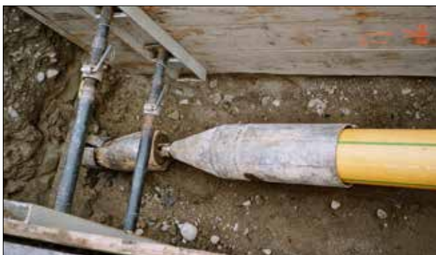
5.29 Pulling head put on the jacketed pipe (incl. jacket thickness)
