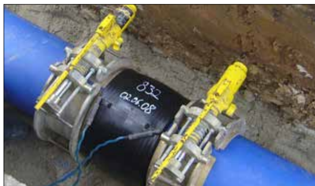
5.80 Re-rounding clamps for EF joints (source: +GF+)
