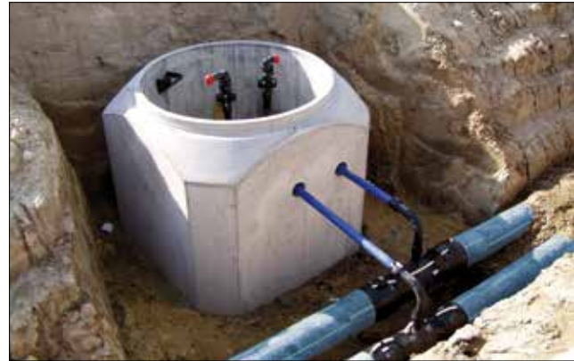
5.79 Tapping fittings for manhole connection
