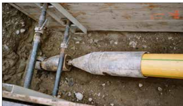
4.24 Pulling head put on the jacketed pipe (incl. jacket thickness)
