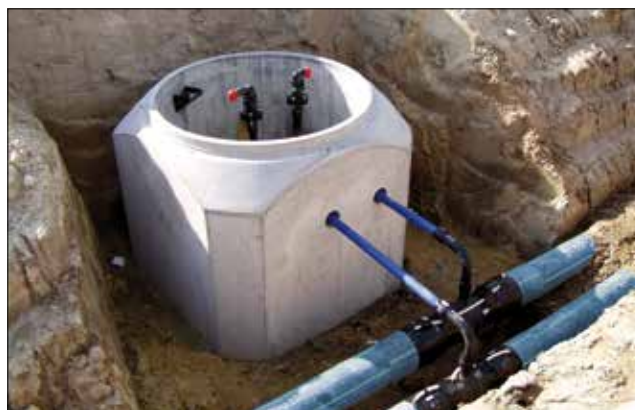
4.56 Tapping fittings for manhole connection
