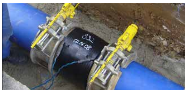
4.57 Re-rounding clamps for EF joints (source: +GF+)
