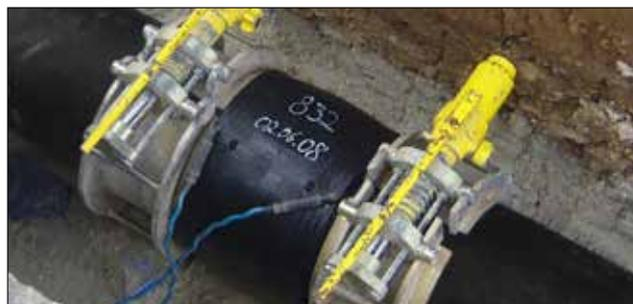
7.38 Re-rounding clamps for EF joints (source: +GF+)
