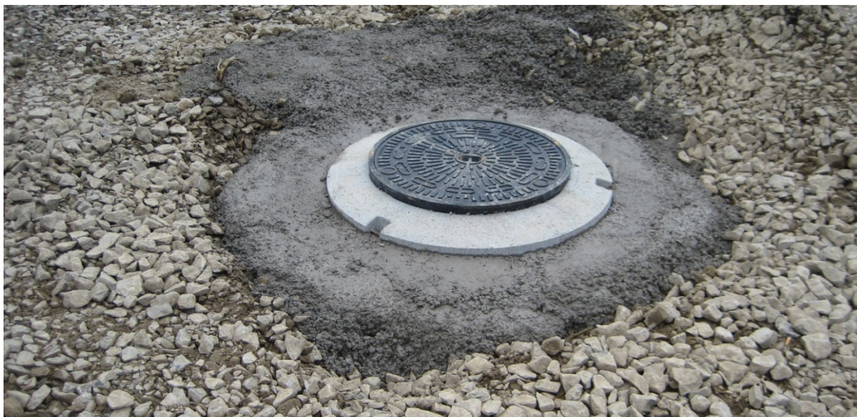
Figure 5: Completed concrete support ring
