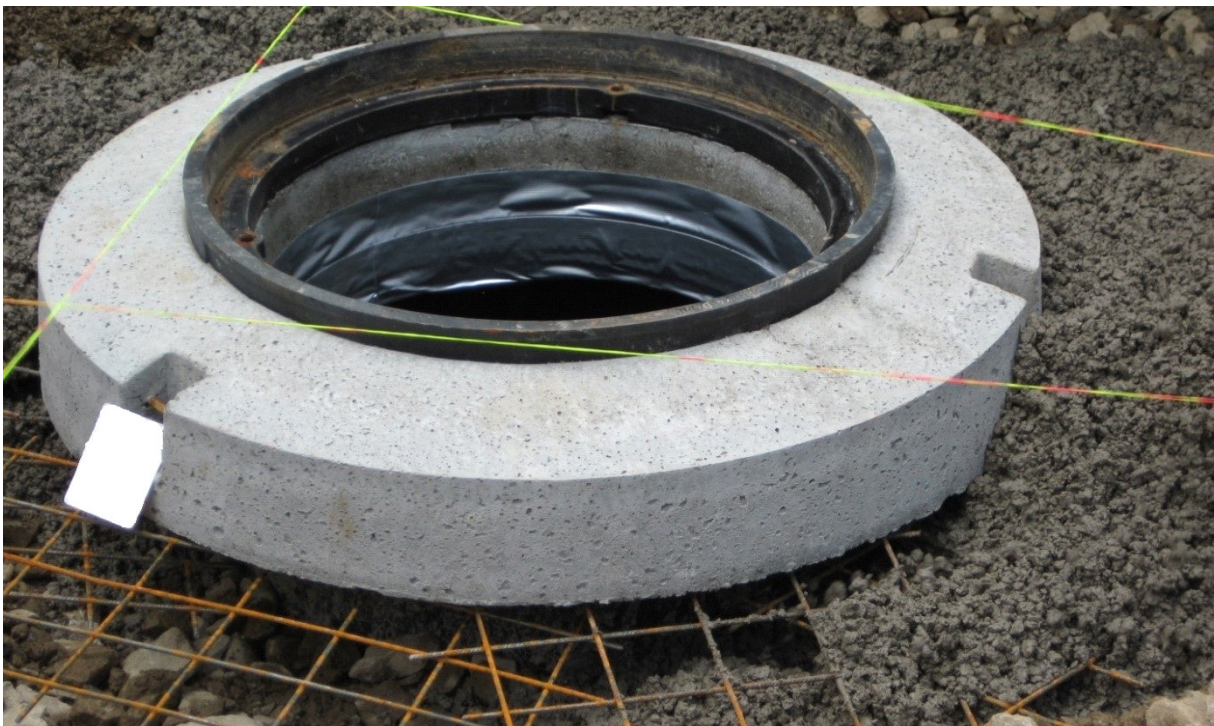
Figure 3: Support of the concrete support ring
