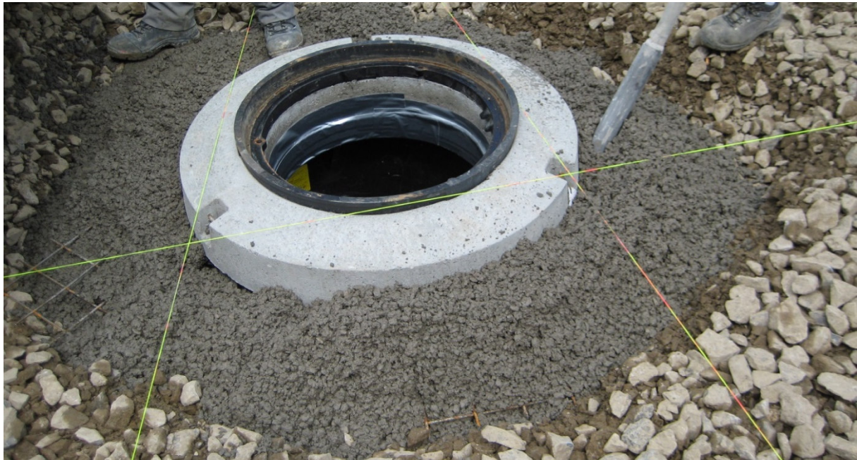
Figure 4: Support of the concrete support ring
