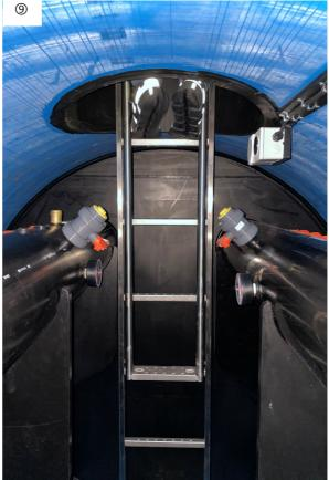
If the dome height is  $\hfill 500$  mm, the dome entrance has a dimension of 630 mm.
