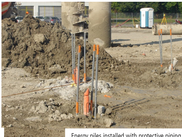
Energy piles installed with protective piping
